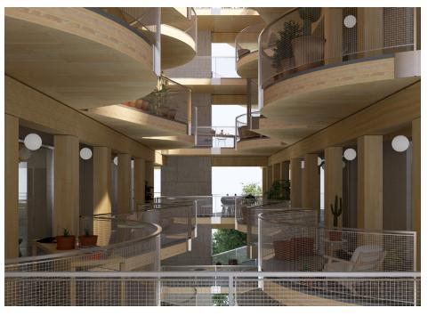
A semi-enclosed and covered atrium space replaces the dark interior hallways of the typical tower. Balconies cantilever off the hallways over the atrium creating additional shared living spaces that are naturally lit from above and from the open ends of the building.
