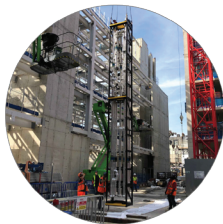
in-situ prefab MEP riser
