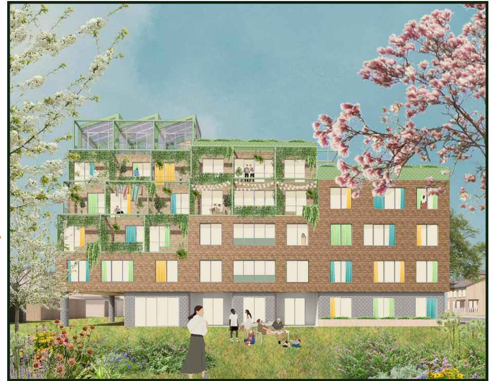
Fig 9. A side view of the building reveals the different layers that make up its geometry: a ground floor Common House full of nooks for gathering, a mass of housing units supported above that steps toward the sunpath, and a verdant layer of roof terraces draped over the top of the building.
